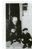
Dad and I on the stoop on the south side of the store. I used to sit here many times watching the trains come and go and the traffic move up and down 7th Avenue.
