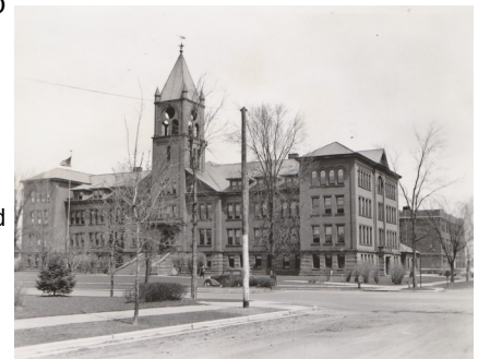
Ashland High School at Ellis Avenue between 10 th and 11 th Streets.
