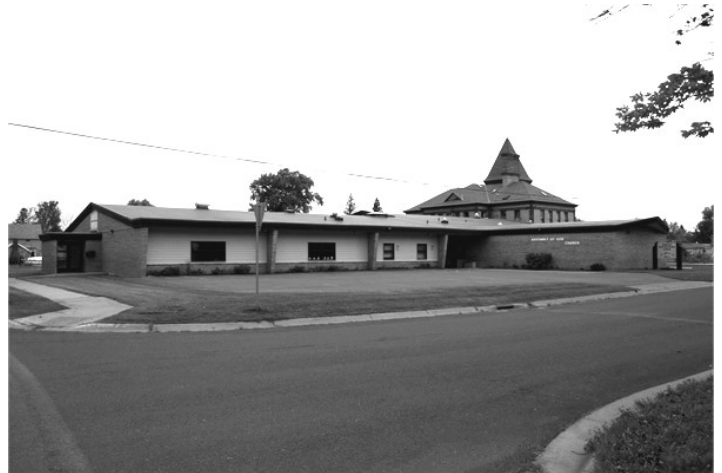
Gymnasium and classroom additions to the back of Wilmarth School.
