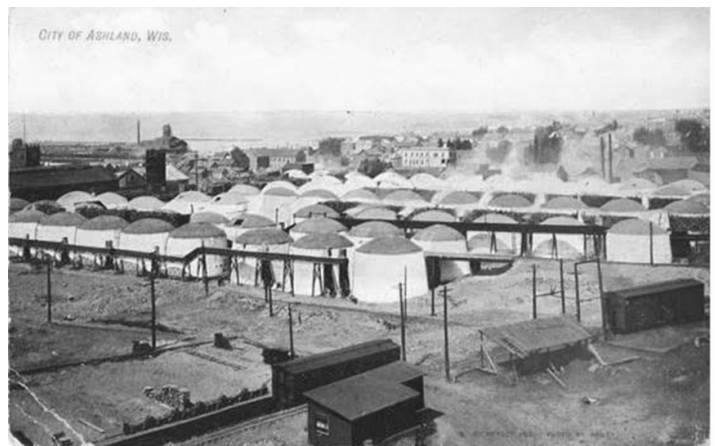
Charcoal kilns at Ashland Iron and Steel, the largest charcoal iron furnace in world.
