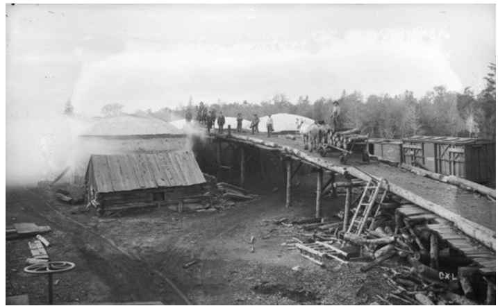
Charcoal kilns at Saxon Wisconsin in 1895. Note the railroad cars adjoining the kilns, with the tops of other kilns in the background.
