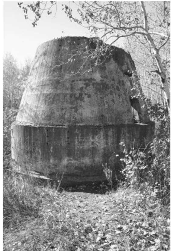
The base of the smoke stack for the Ashland Steel and Iron blast furnace, located on Sanborn Avenue.
