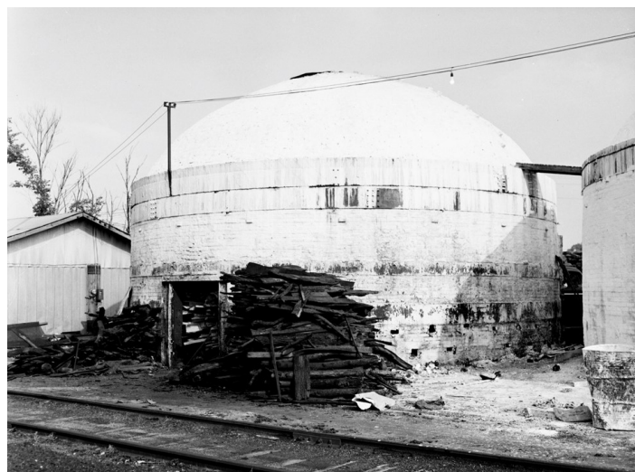
A circular charcoal kiln with a beehive type top, similar to the kilns along Wisconsin's rail lines. Charred slabwood piled in front of the kiln.
